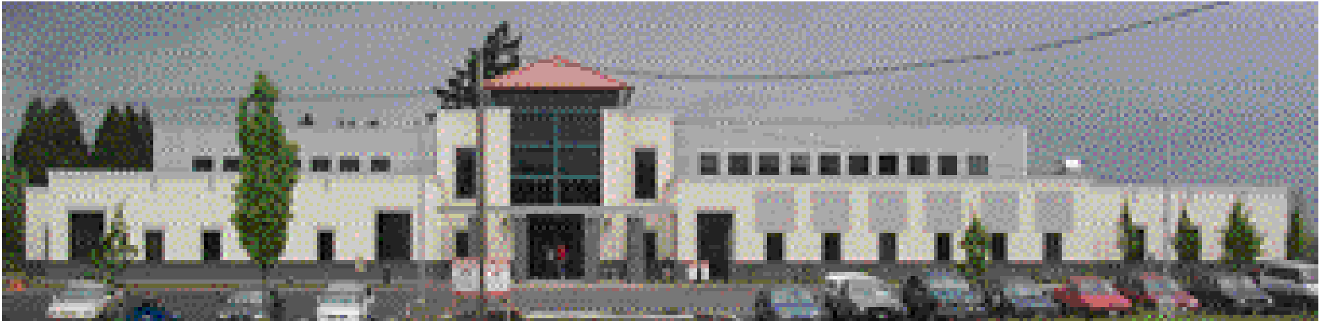
The new shelter at the completion of Phase II.
