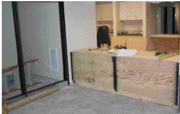
Construction of the cattery area.
