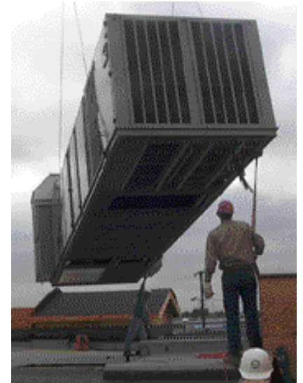
Bringing in the HVAC system for installation.
