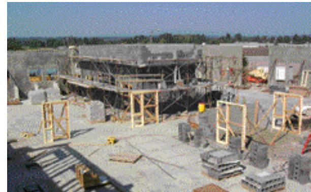
Construction of the kennel area.
