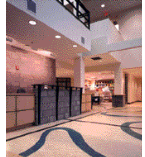
Linoleum flooring in the lobby Photo by: Ed Hershberger
