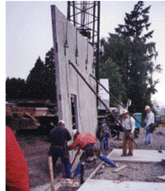
Concrete tilt-up walls used in the kennel area
