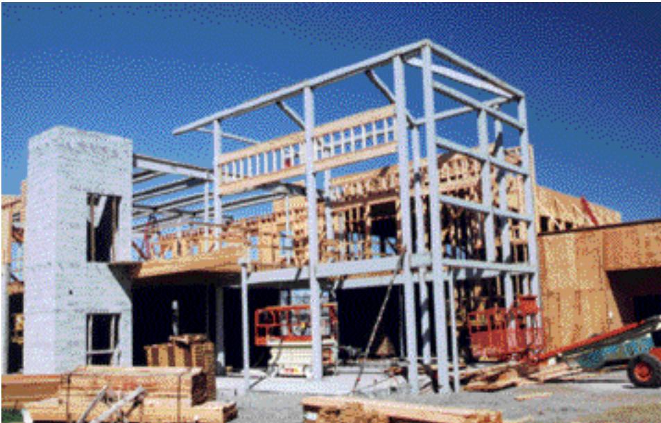
Concrete block, metal, and wood structure of the building front
